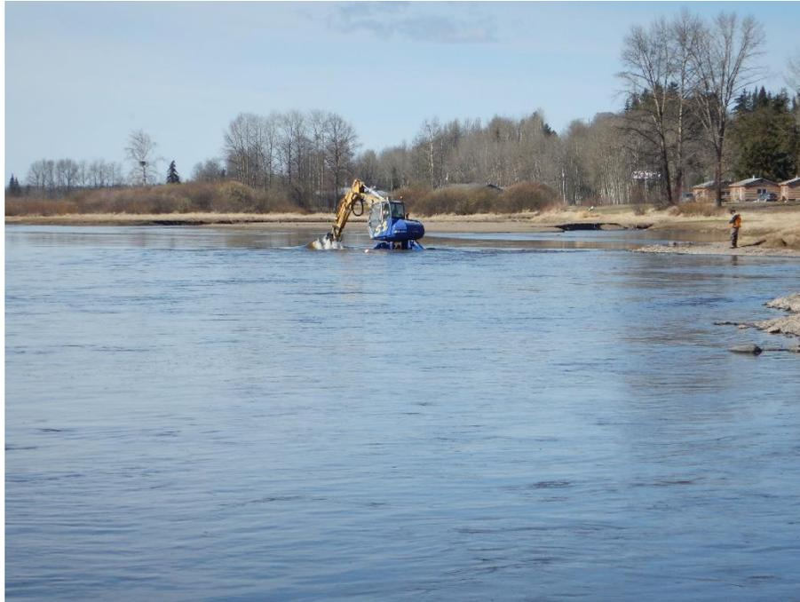
**Figure 4** Excavator beginning the remedial work at the upstream extent of the Lower Patch.
