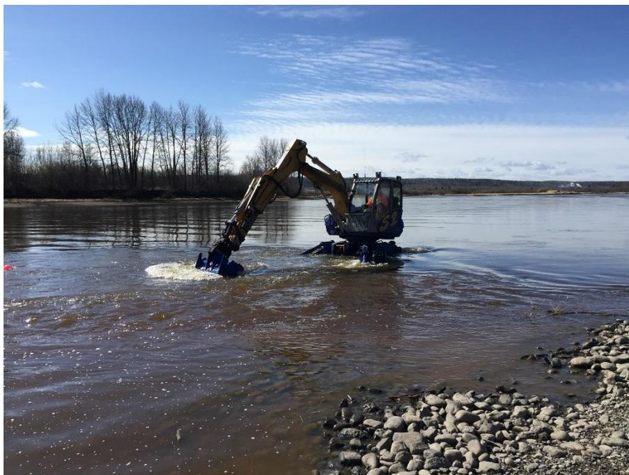
**Figure 3** Excavator with 1.5 m-wide toothed bucket raking and sifting the cobble/gravel bed at the Lower Patch (placed substrate seen along bank).
