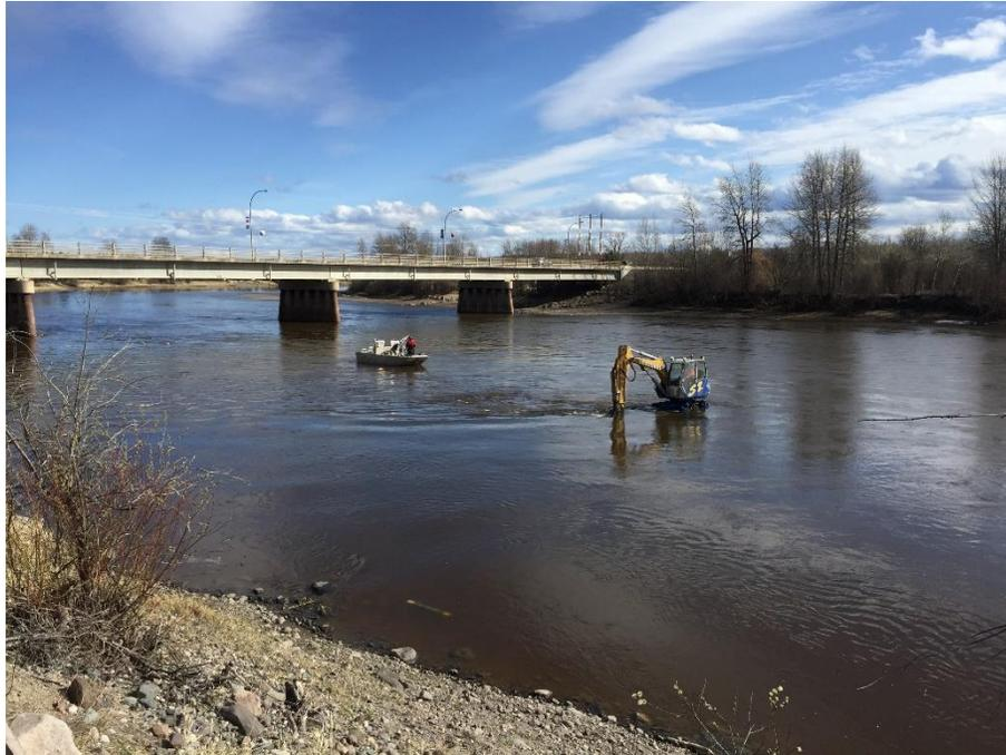
**Figure 7** Sampling bedload sediment transport directly downstream of excavator.
